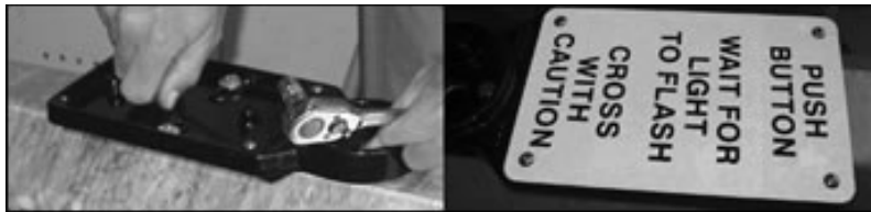
Figure 6.10: Push-button plate (left) and sign (right)
